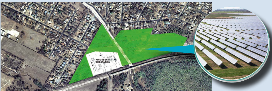
The Kingsbery substation community solar project.
